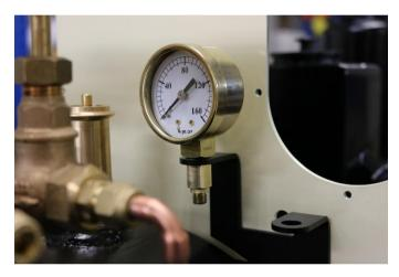
Fit the pressure gauge to the bracket, the union nut acts as the locking bolt to secure it in to place, the pressure gauge must have PTFE tape on it before fitting to ensure a good sealed join.
